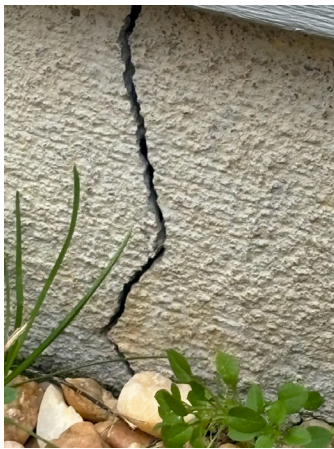
Crack – Left, Middle (Close to 1/4 inch)
