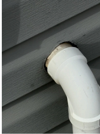
Non Sealed Opening Around Condensation Line (Right, Bottom)
