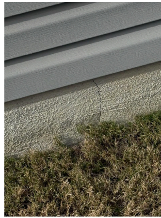
Hairline Crack – Right, Back
