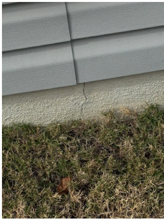
Hairline Crack – Right, Front
